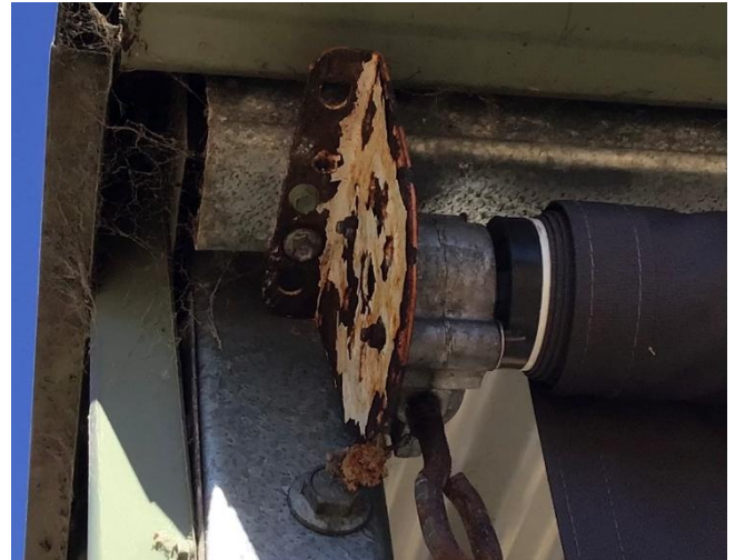
Figure 2 Showing TEK screws to be removed
