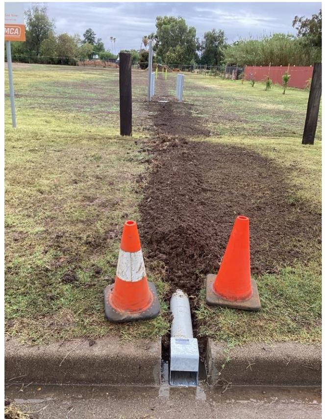
Figure 5 Drainage works showing the final connection to Chandos St kerb and pits in the background
