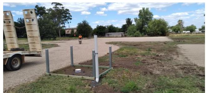
Figure 5 Form work for dump point at Gunnedah
